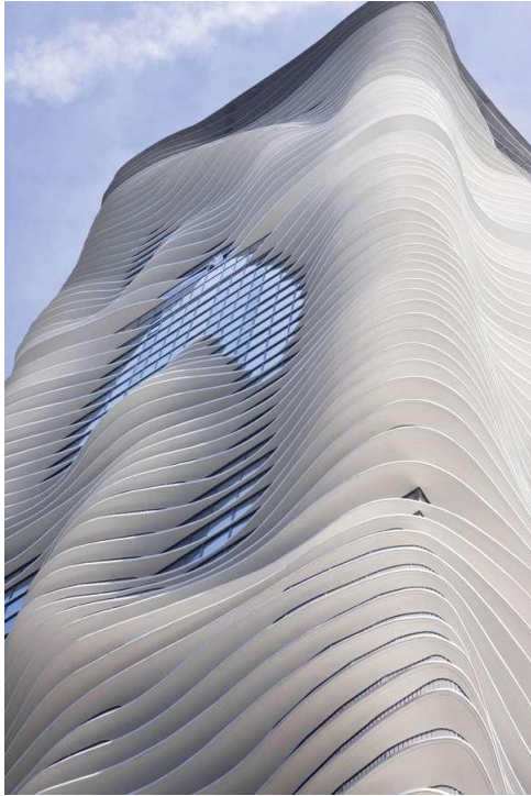
Aqua Tower, Chicago, designed by Jeanne Gang, 2010.
